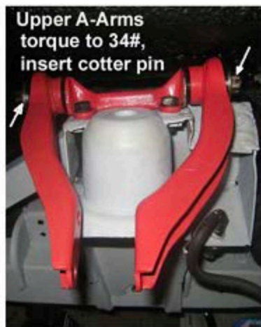
UPPER A-ARM INSTALLED
